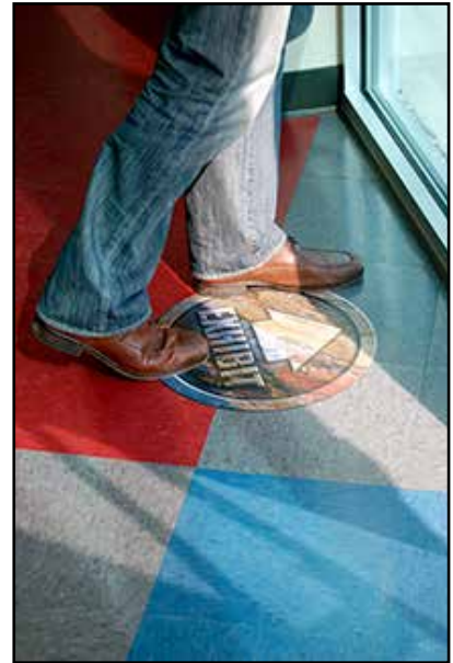
Lambda Vinyl Flooring profile cut and applied to floor.
